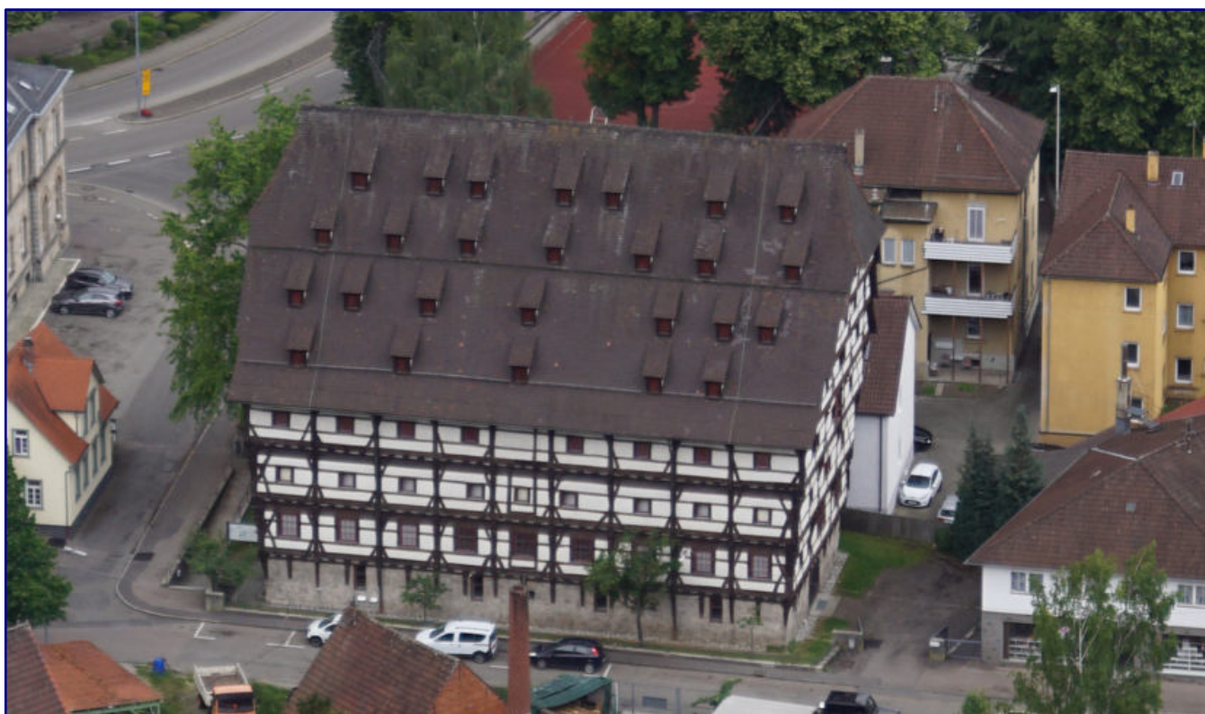
The last location of the former Geislingen depot now houses the sidings for two class 185 banking engines (photo above). The Alter Bau ("Old Building"), a large granary dating from 1445/46 (photo below), now houses the municipal museum, which has a 28-metre-long model railway layout on one gable end.
