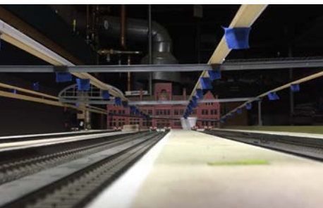
5. Test fit subframe to platforms
